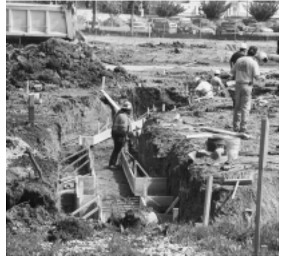
Library construction is on time and on budget. Here footings are placed along the south side. For the latest construction pictures, visit www.elmhurstpubliclibrary.org .
